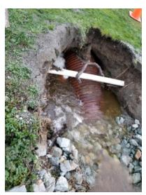
This temporary repair was accomplished using a 10-foot-long section of steel culvert pipe molded to fit inside of the existing structure to reinforce and stabilize the side walls and entrance opening. Sometime this summer Island County will replace the entire culvert with a new culvert drain pipe.
